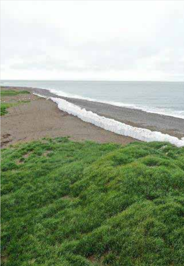
Super sack protection looking southwest
