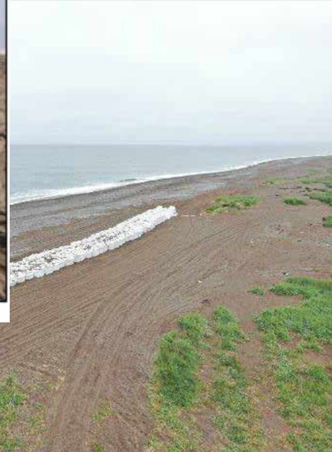
Super sack protection looking northwest
