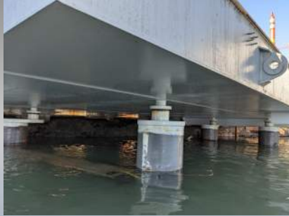
Current Pier Pile Connections
