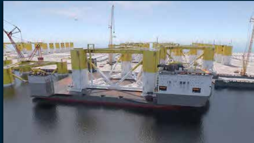
LOADOUT ONTO SEMI SUB
