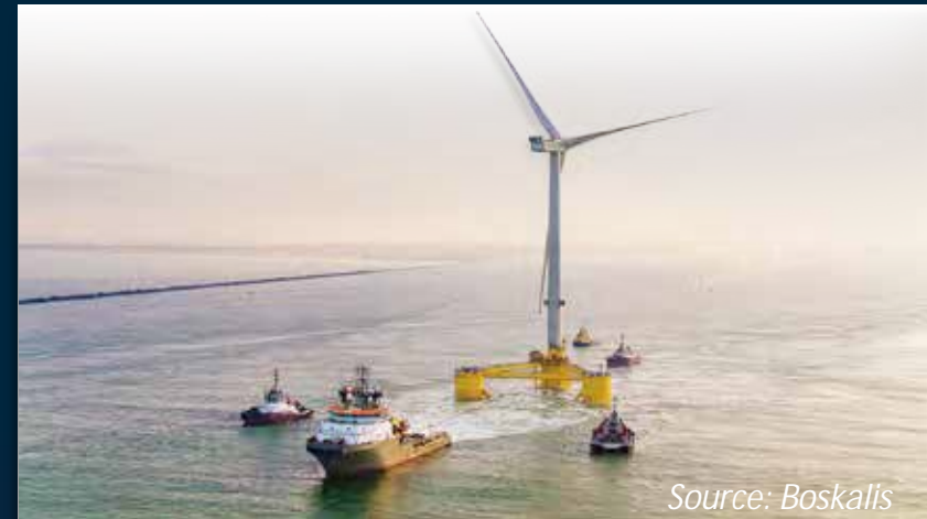
TOW OUT TO INSTALLATION SITE
