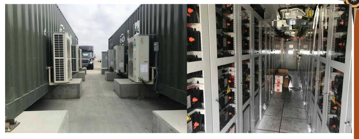
Each BESS has 1.2 MWh energy storage with a max output of 500kVA, 480 VAC Three Phase Lithium Ion
